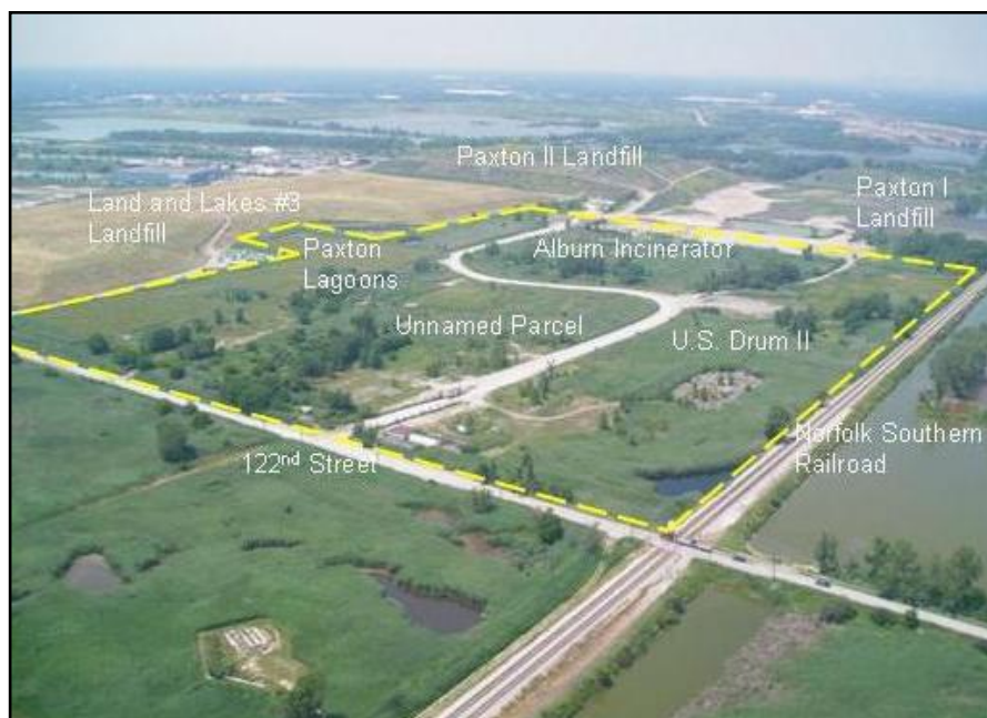
Figure 2 – Aerial Photograph of the LCC Site
